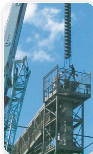
Quick and simple assembly of an endless chain strand
